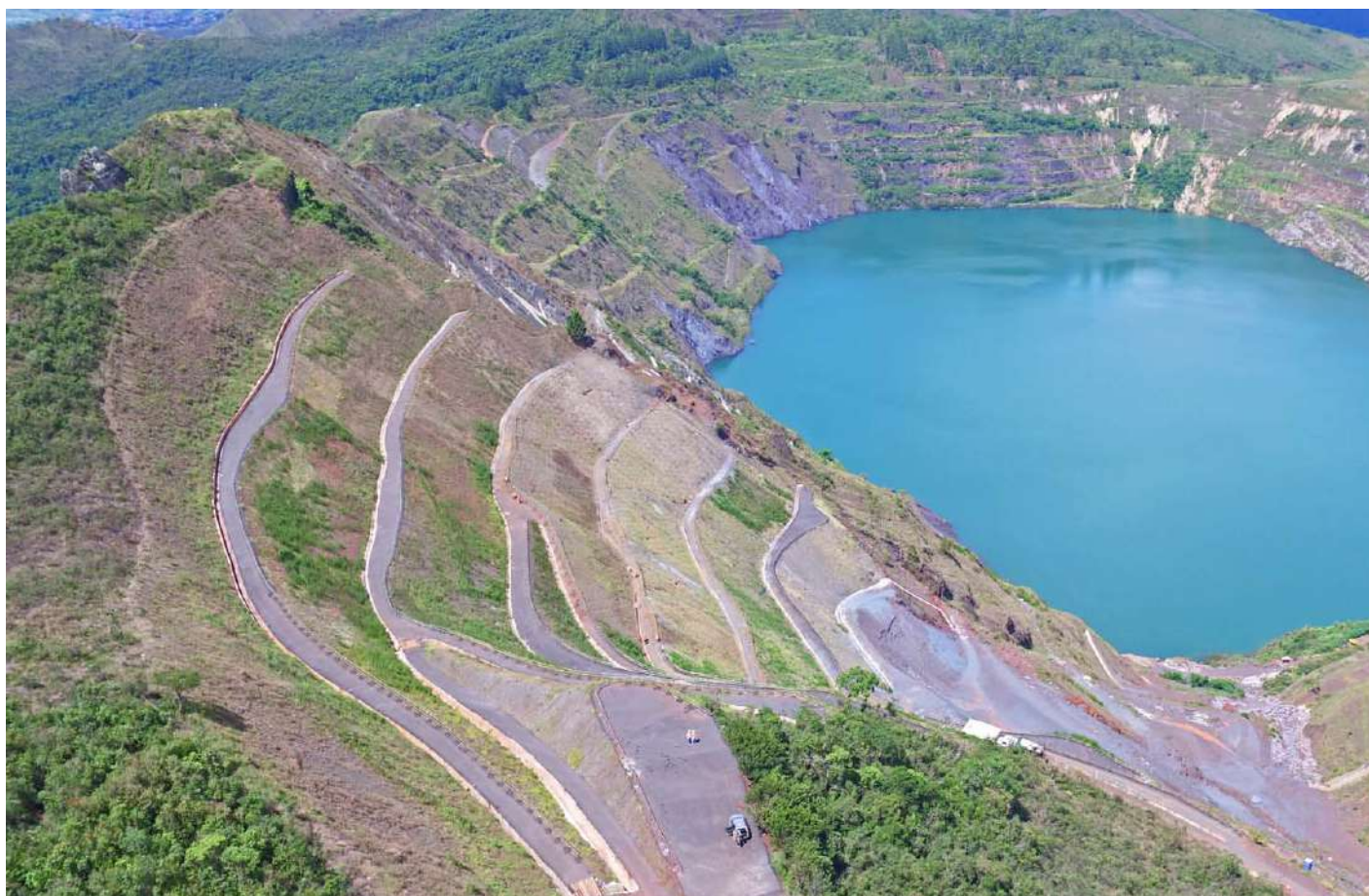
Slope stabilisation in the West Put Sector - Águas Claras Mine - Nova Lima - Mine - Nova Lima - Minas Gerais | Brazil
