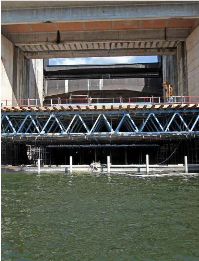
Formwork and Pre-stressing Operations Centre Construction of a platform for geotechnics works Crestuma-Lever Dam | Portugal
