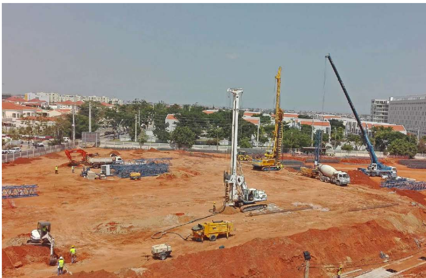
Indirect foundations of the Talatona 2 building - Luanda | Angola
