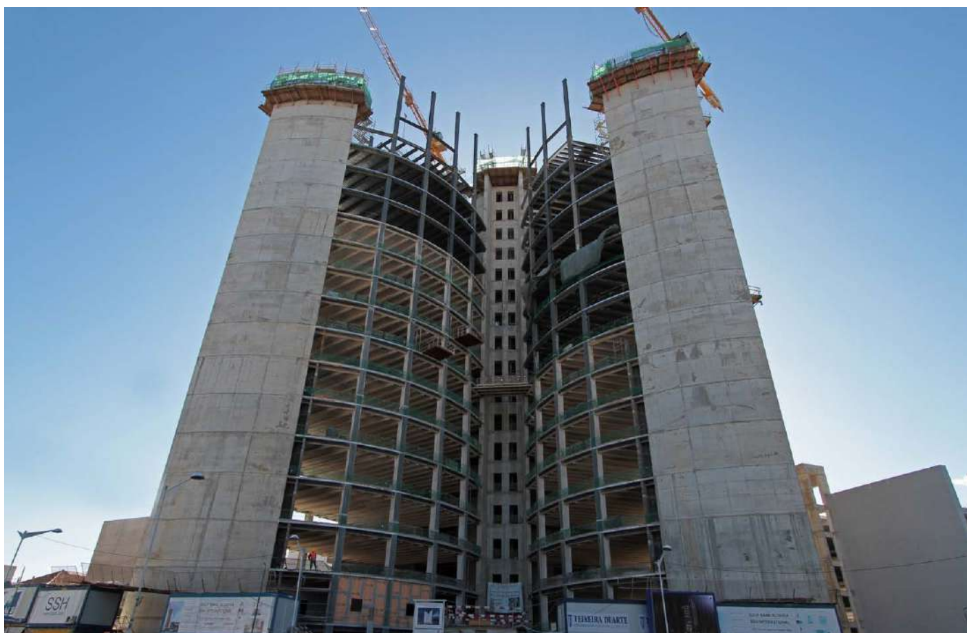
Construction of the new headquarters of Gulf Bank Algeria - Algiers | Algeria
