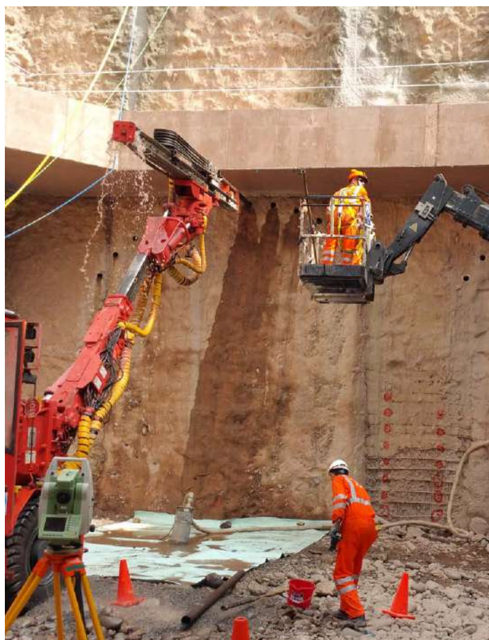
E.P.O.S. – Empresa Portuguesa de Obras Subterrâneas, S.A.: Excavation and cladding of galleries – Lima Metro Lima | Peru
