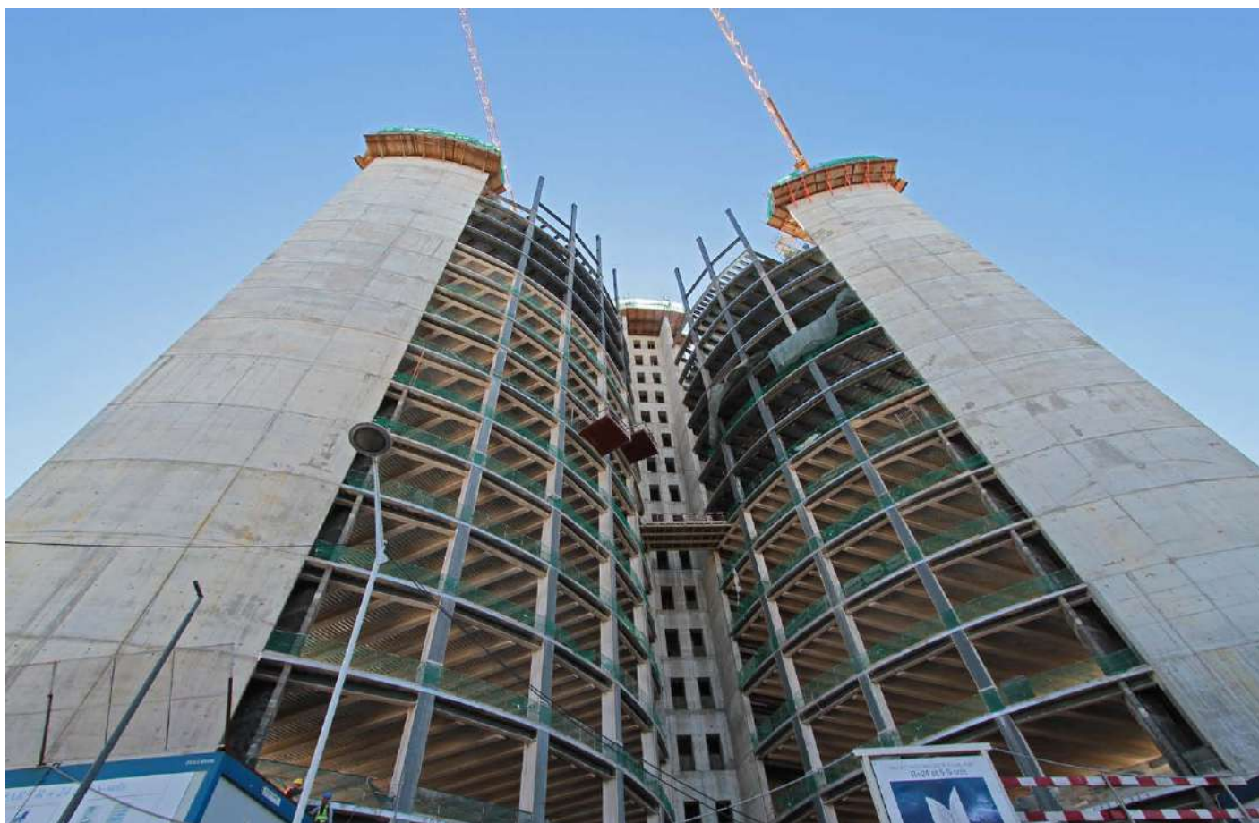
Assembly of metal structures - New headquarters of Gulf Bank Algeria - Algiers | Algeria
