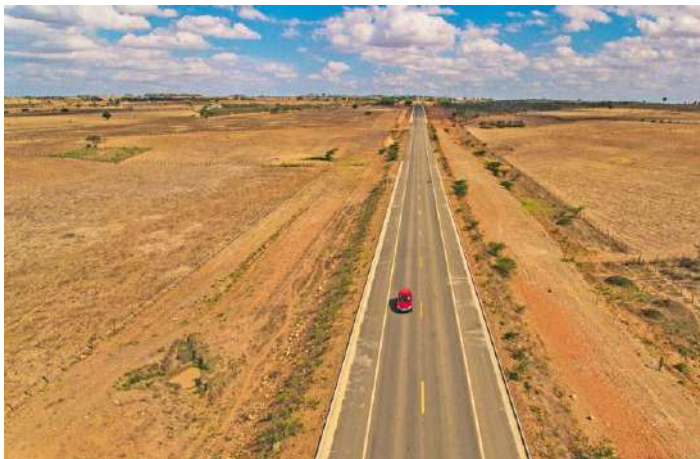
Modernisation work on the Thenia/Tizi-Ouzou line – Bordj Manaiel Station Boumerdès | Algeria Construction of Highway BR 235 / BA – Coronel João Sá Bahia | Brazil
