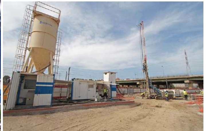
EMPA S.A. Serviços de Engenharia Foundations for the São Luís do Maranhão Terminal | Brazil Teixeira Duarte Algérie, SPA Micropiles and jet grouting – Oued Ouchayah | Algeria
