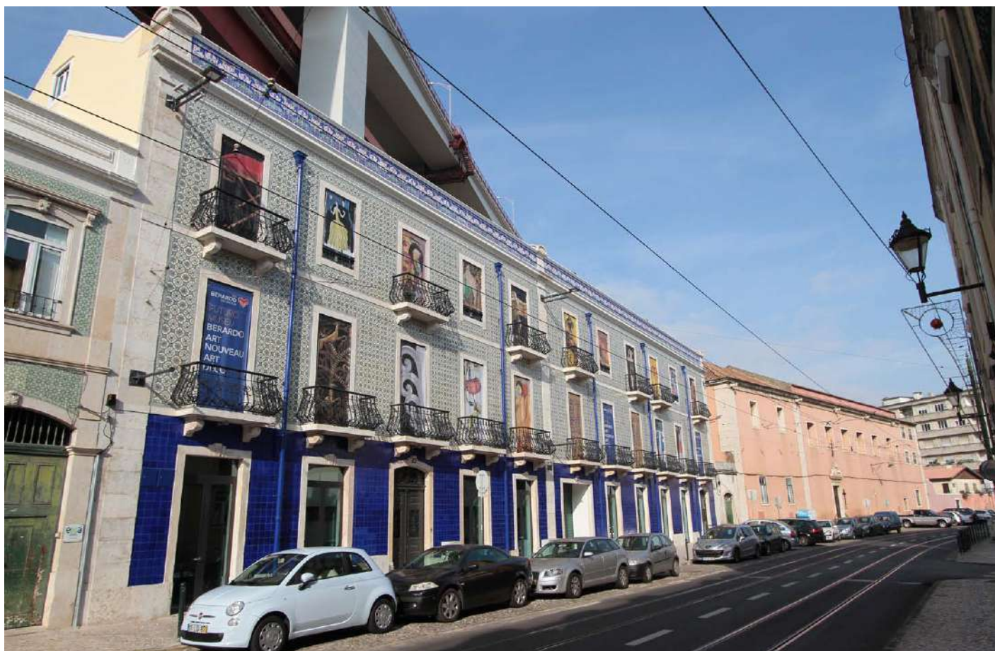
Conservation and alteration of external frontages - Lisbon | Portugal
